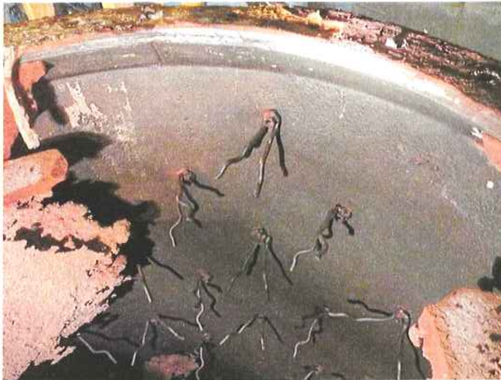
This is a close-up within the scrubber showing the eroded refractory lining. MSD staff have temporarily repaired this.
