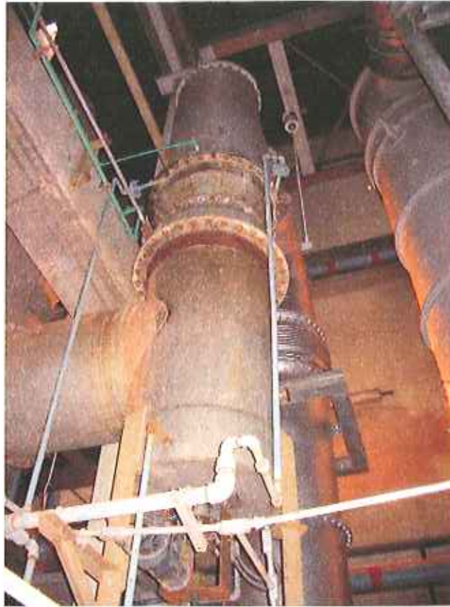
The Venturi Scrubber is shown above. Note that the piping is 3-feet in diameter.
