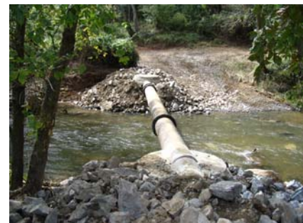
Example of sewerline crossing creek
