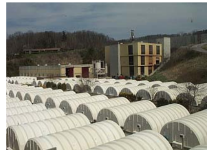
View of RBCs and Incinerator Bldg.
