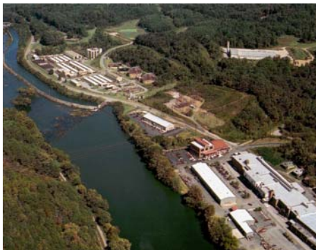
Aerial view of Metropolitan Sewerage District
