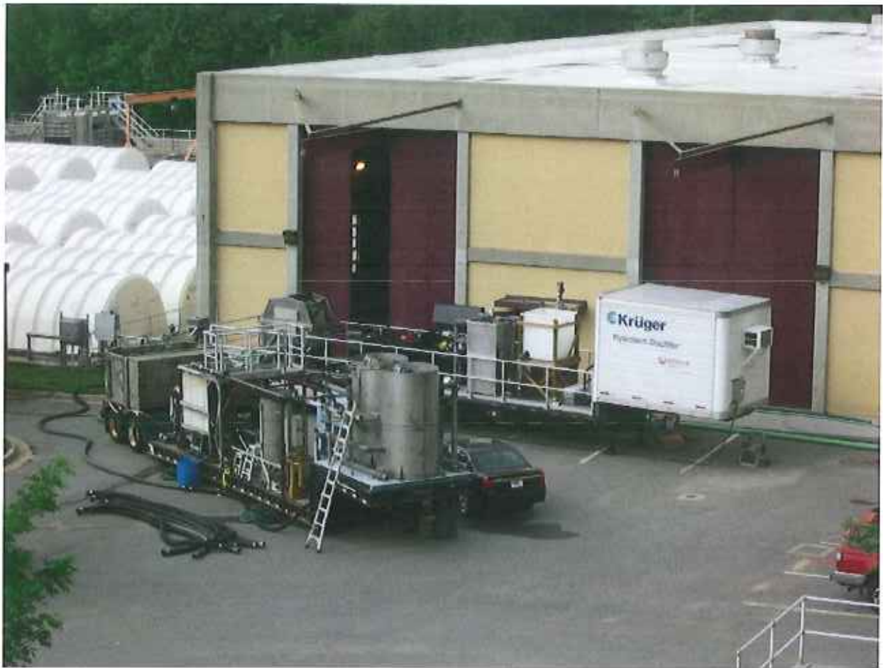
~ Side-By-Side Pilot Testing (May 2007) at the MSD Final Microscreen Facility ~ On the left is the Aqua-Aerobics AquaDisk System, on the right is the Kruger Hydrotech Diskfilter.
