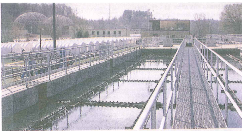
Seeking clarity: First, MSD treats the raw sewage with microbes, then lets the solids settle to the bottom of these ponds.
