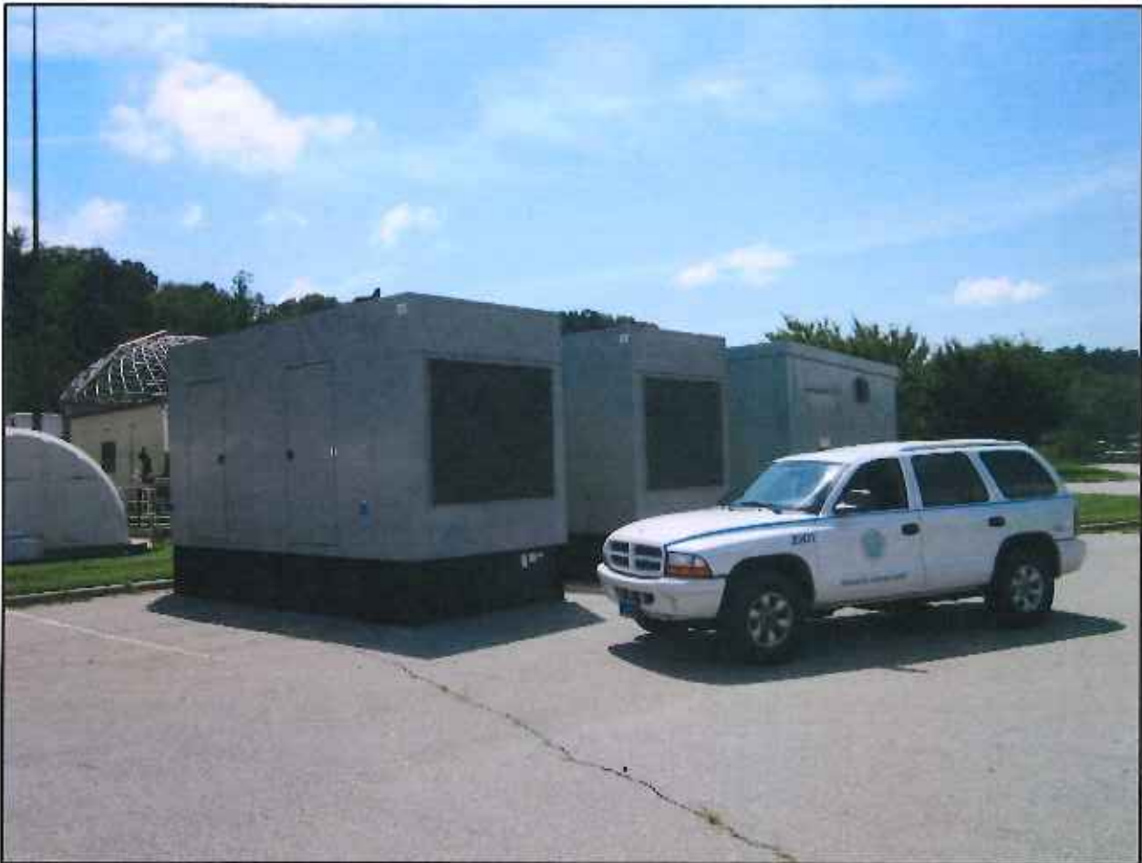
Each of the two gensets generates up to 1 megawatt. The new switchgear is in the rear. Note the vehicle for scale.
