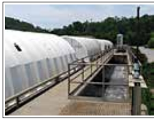
Rotating Biological Contactors
