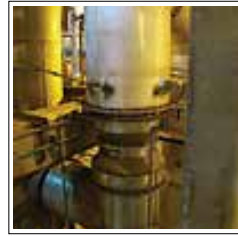
Ash Removal Venturi Scrubber
