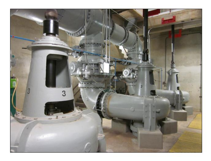
Three 400hp influent pumps - the largest pumps in MSD's system. Typically, only one pump is needed to maintain *all* wastewater flowing through the plant.
