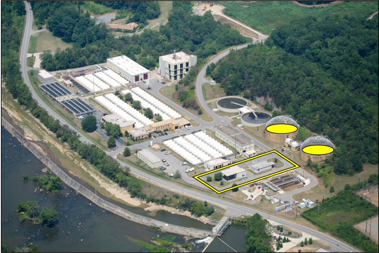
Plant Aerial Photo showing Project Areas
