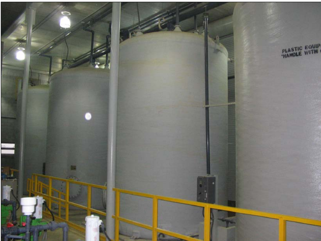
This is the interior of the facility, showing the Four 15,000 gallon Tanks.
