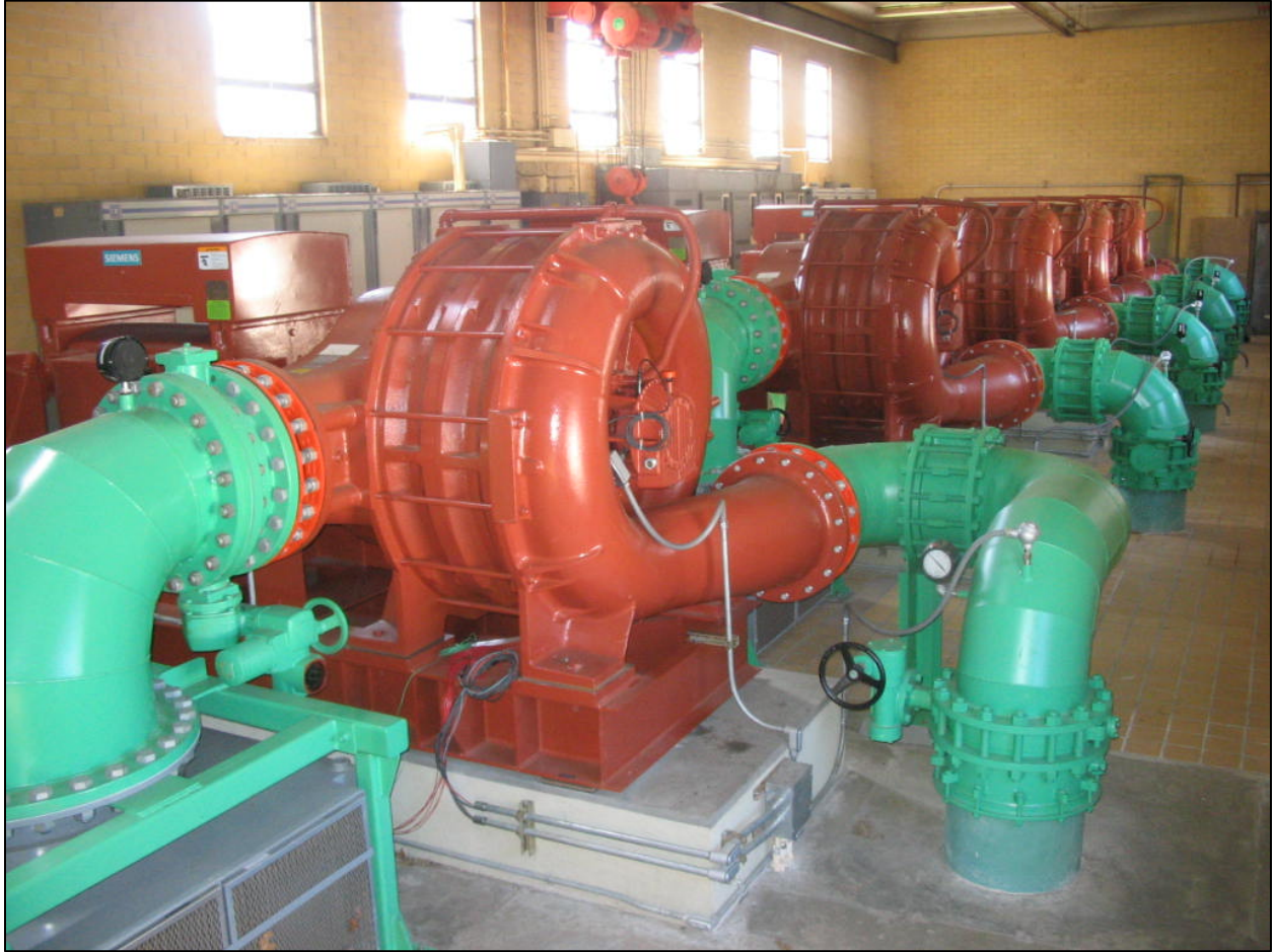
This picture shows the blowers, which provide large volumes of air to rotate the RBC's.
