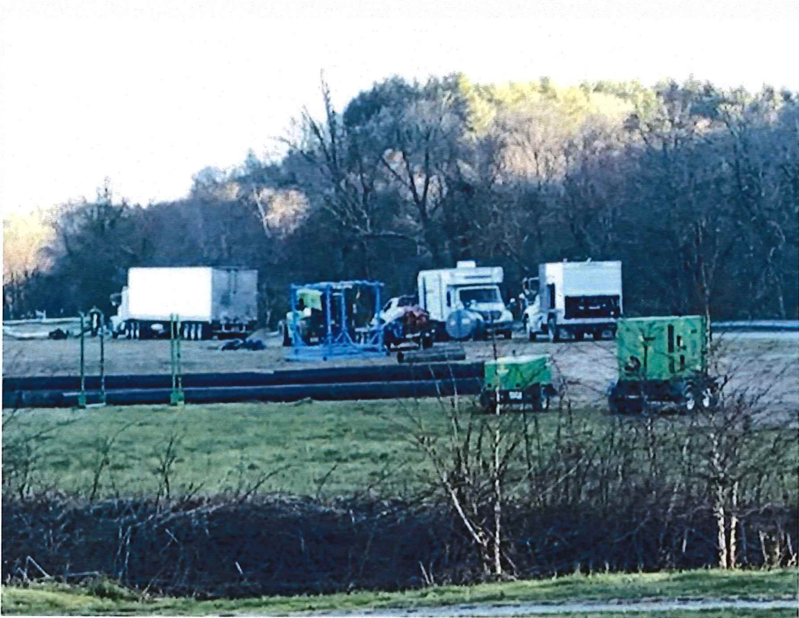
The Metropolitan Sewerage District is putting a new liner in a 36-inch sewer line that runs along the French Broad River through the Biltmore Estate. The large black line above ground is a temporary rerouting of the main line. (Photo: John Boyle/jboyle@citizen-times.com)
