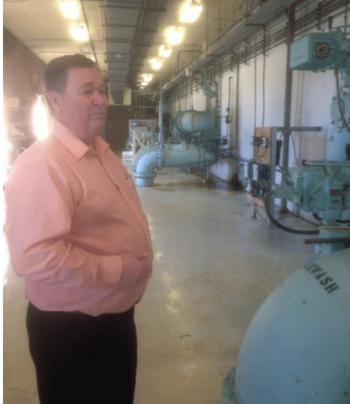
Terry Shelton, the director of environmental services for Eden, explains the treatment process at Eden's drinking-water plant. Photo: Gabe Rivin
