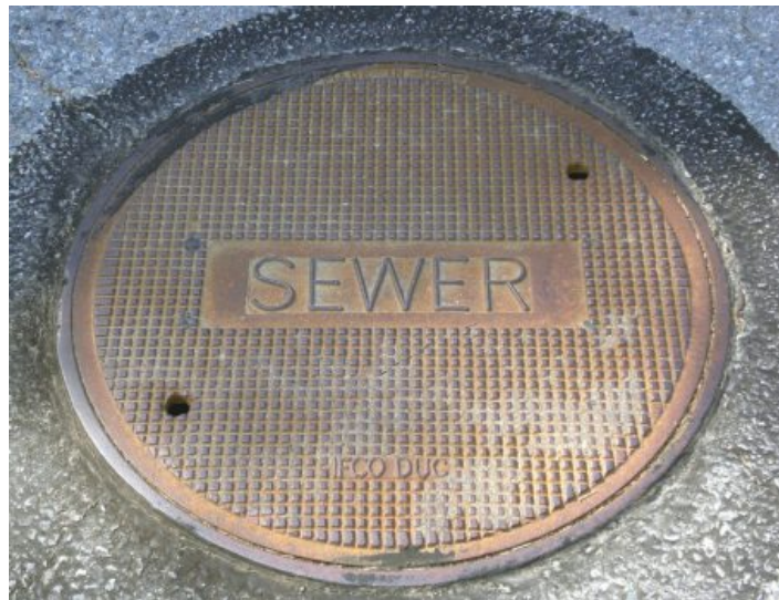
A cover for a municipal sewer access point. Municipal sewer systems transport human waste from homes and businesses, and treat it in centralized wastewater plants. But most folks don't think about where it all goes after they flush. Photo courtesy Wikimedia Commons
