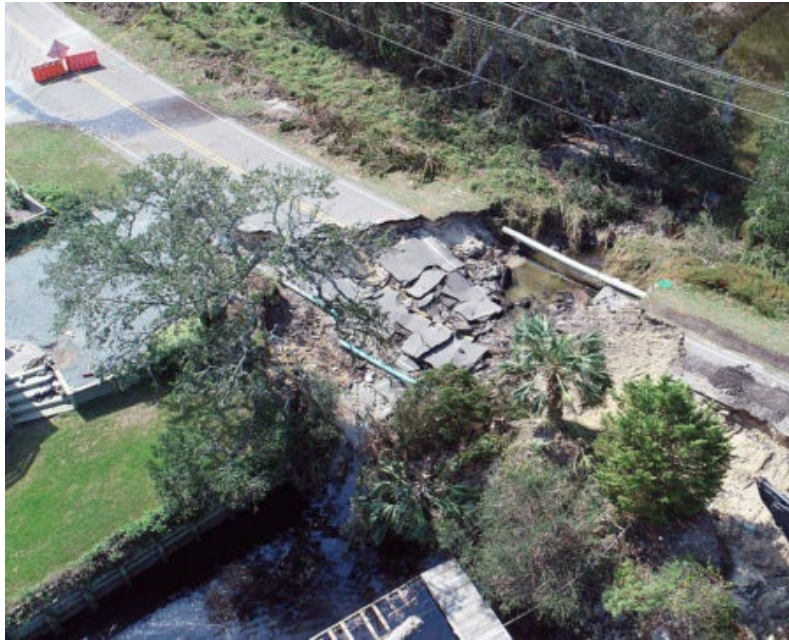
A view of the washout on Middle Sound Loop Road in Wilmington on Sept. 20, 2018 with pipes exposed. The challenges facing water system managers after storms come from both overflows and damage to infrastructure. Photo courtesy: NC Department of Transportation
