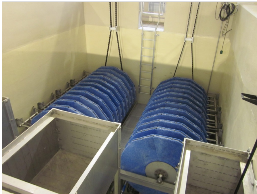
This picture shows two filters and the filter media (blue). There are sixteen filters.
