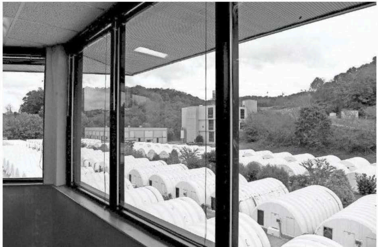
Rows of rotating biological contactors work as a step in the process of treating Asheville's wastewater at the water reclamation facility of the Metropolitan Sewerage District on Oct. 9, 2018. The facility has 152 rotating biological contactors. ANGELI WRIGHT/CITIZEN TIMES
