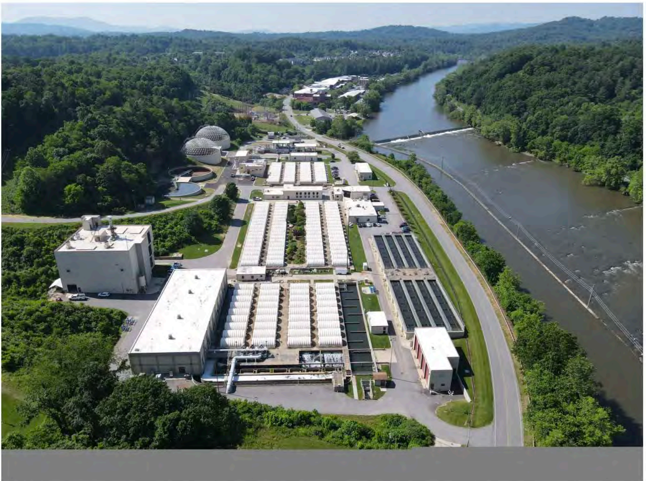
The Metropolitan Sewerage District of Buncombe County's facility in Woodfin processed 8,531 dry tons of sewage sludge in its last fiscal year, a spokesman says. // Photo credit: MSD
