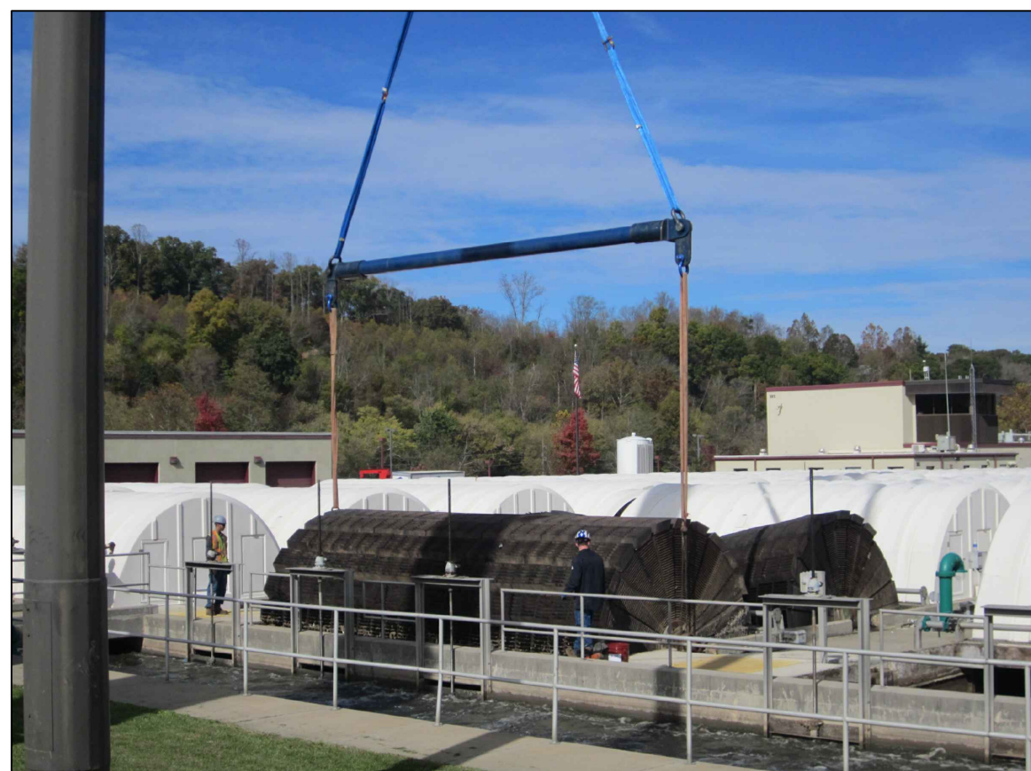
REMOVAL VIA SPREADER BAR
