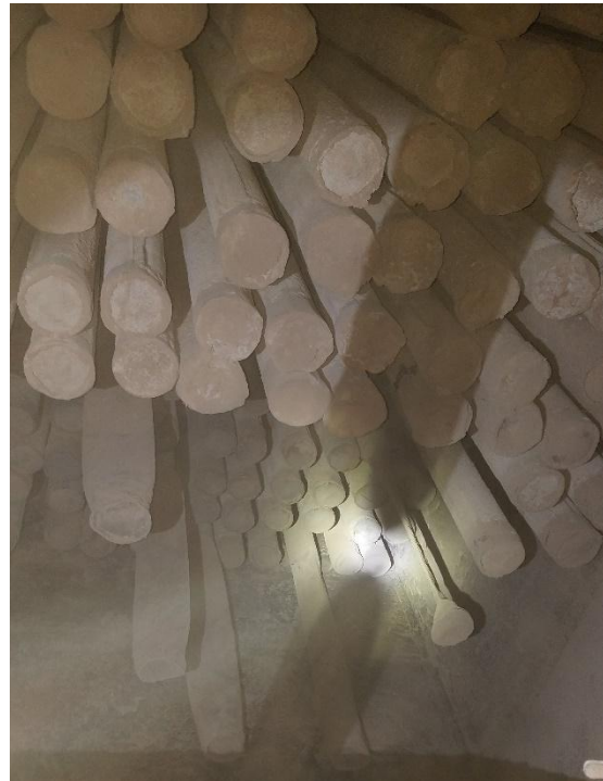
Figure 12. Carbon injection bag house
