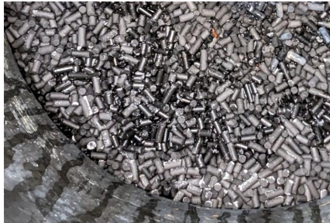
Figure 9. Activated carbon pellets in an adsorber
